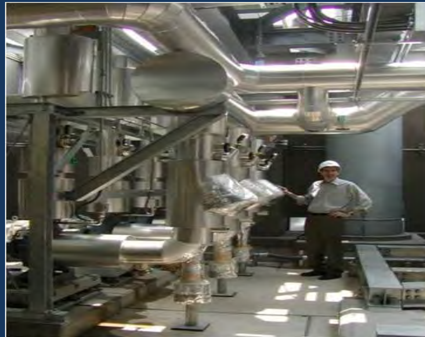
Piping to cooling towers
